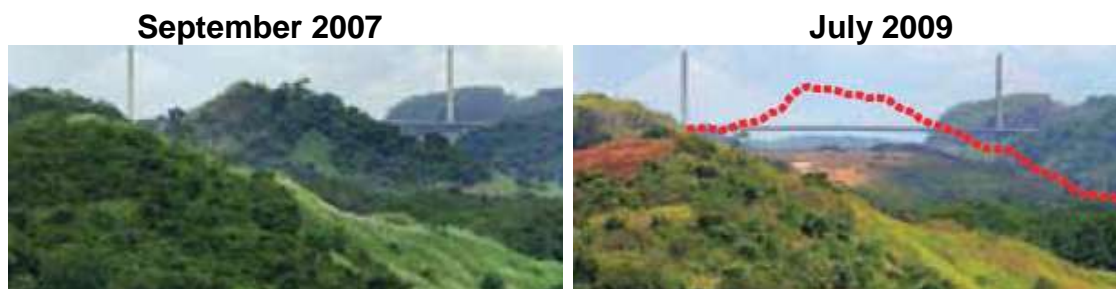
Figure 22: Paraiso Hill Excavation for the Pacific Access Channel, 2007 and 2009
